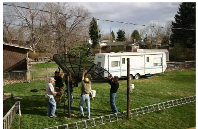
The tower safely down, the team remounts the satellite dish.
